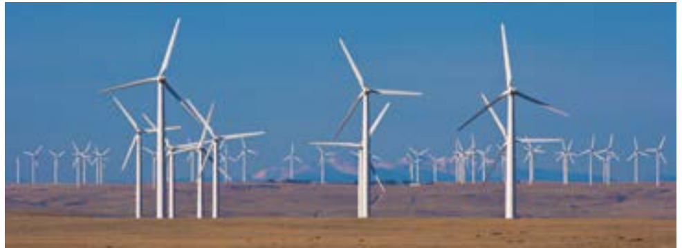
Turbines at BP's Cedar Creek wind farm in Colorado – wind was one of the three fastest-growing forms of new power generation globally between 2010 and 2015.
