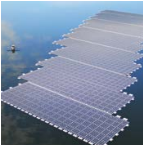
Europe's largest floating solar farm – at the Queen Elizabeth II reservoir near London – built by Lightsource BP.
