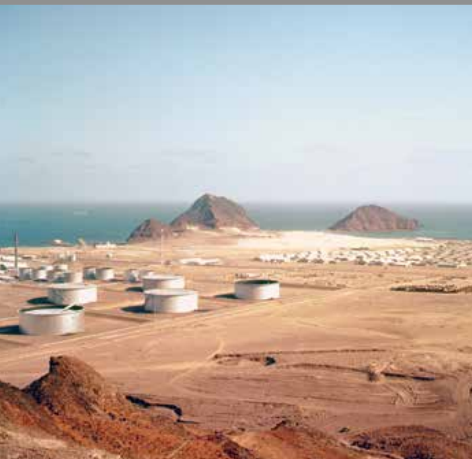
Above: BP's Little Aden refinery in Yemen, located adjacent to the eastern approaches to the Red Sea.
