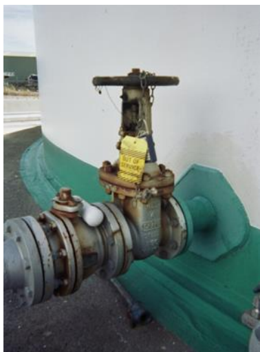
Figure 1: Single Valve Isolation with Lock and Tag
