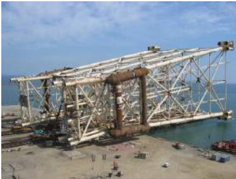
Figure 5.9 DWG-DUQ Jacket During Loadout
