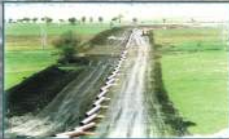
Top soil segregation and management
