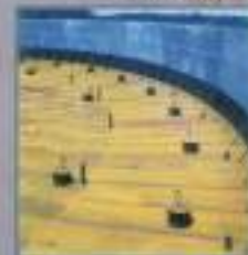
FLOATING ROOF FOR VOC CONTROL
