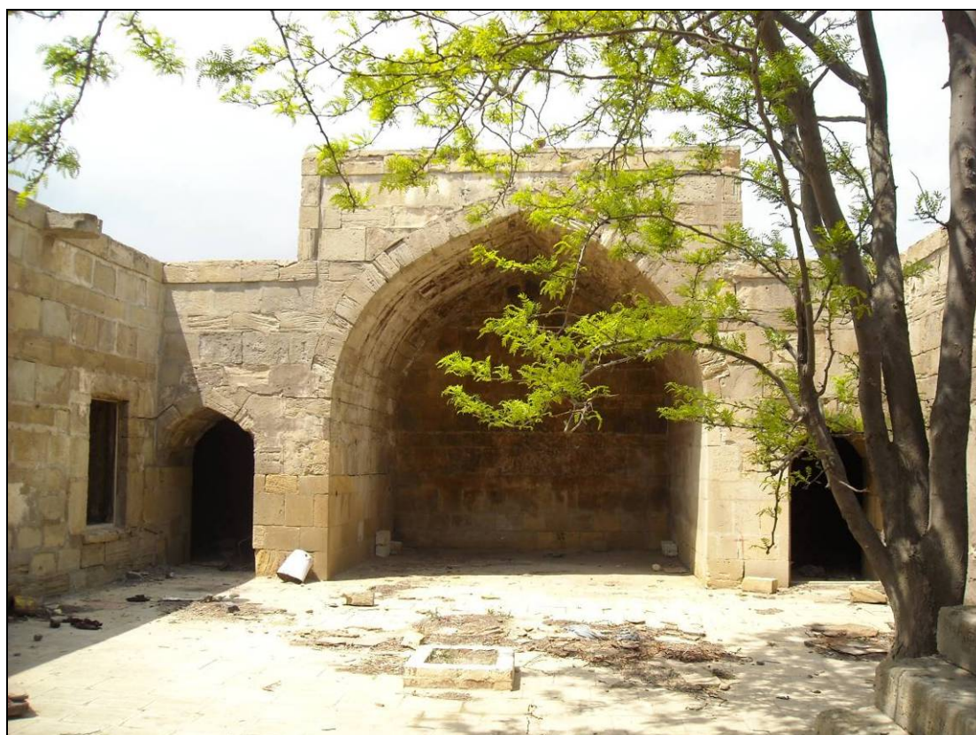
Figure 6.15 Courtyard Interior of the Caravanserai
