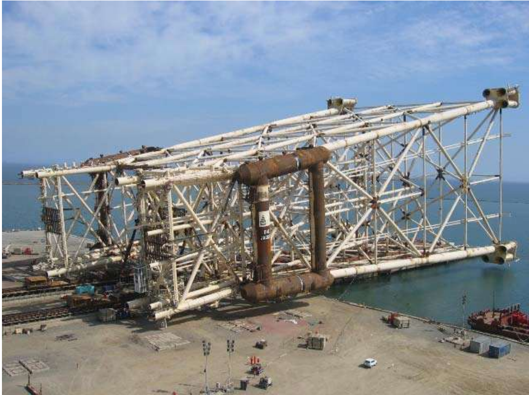
Figure 5.7: DWG-DUQ jacket during loadout
